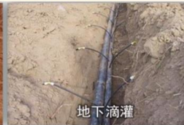
Subsurface drip irrigation
