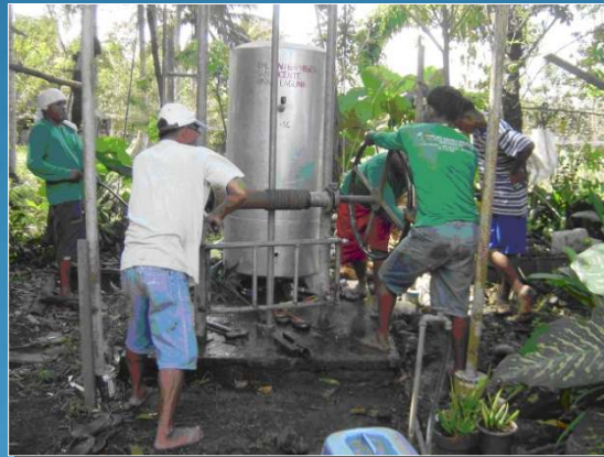
Deep well rehabilitation process
