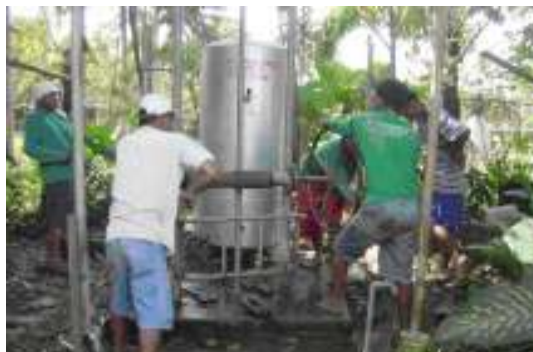
Figure 13. Deep well rehabilitation process
