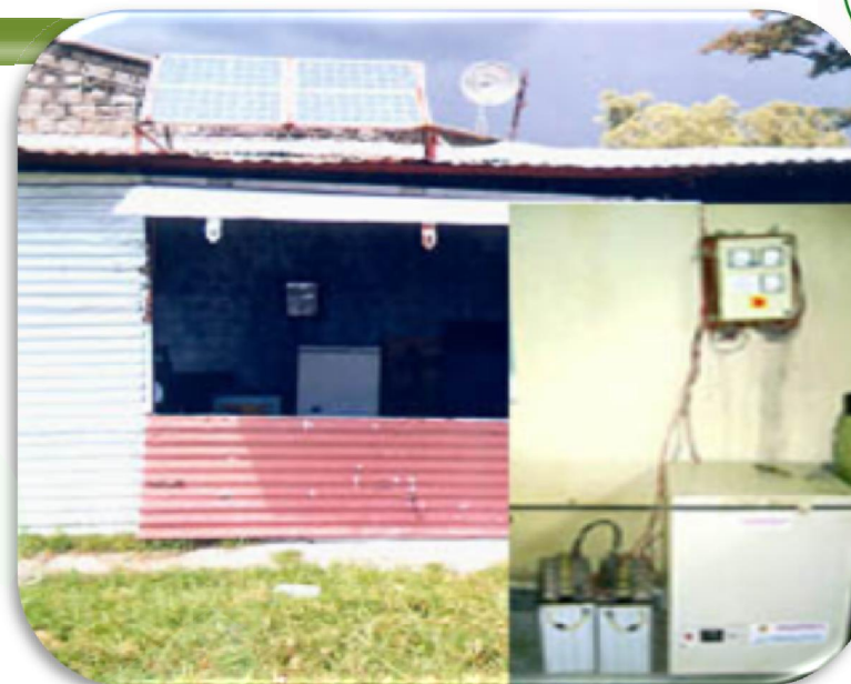
Solar Refrigerator installed at Veterinary laboratory of CSKHPKV Palampur
