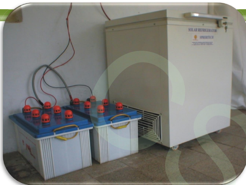
Solar Refrigerator installed in a veterinary clinic near Anand
