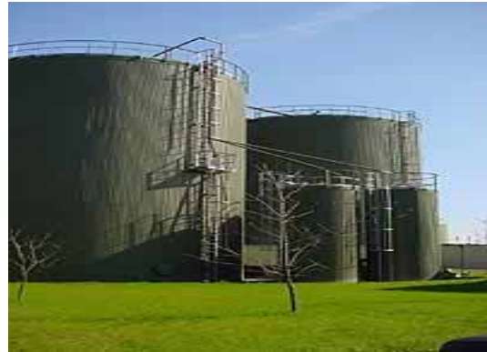
Photo 4: Anaerobic digesters
