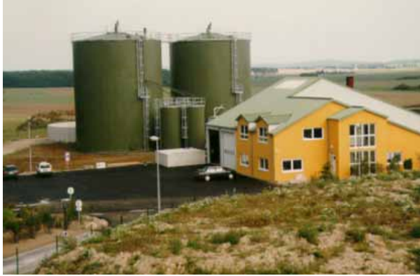
Photo 3: Biogas plant Riegen
