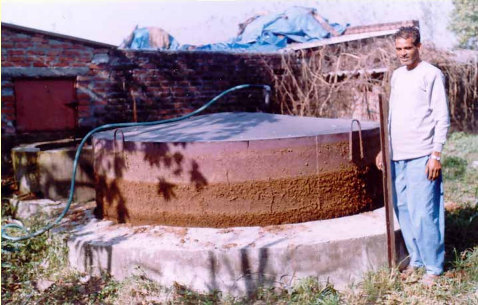
**6 m<sup>3</sup> Pant Tarai Biogas Plant
