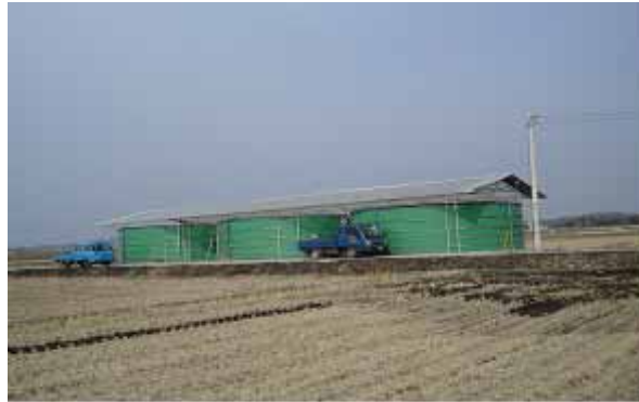
Fig. 10 Liquid manure storage container
