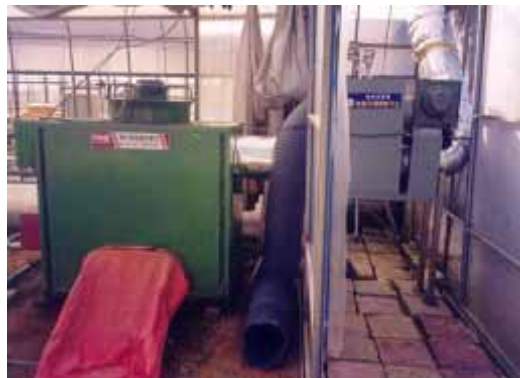
Fig. 5 Exhaust heat recovery system for warm air heater
