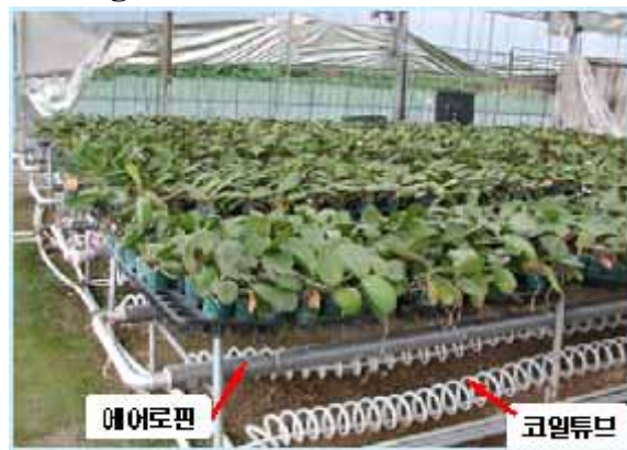
Fig. 3 Coil tube hot water heat exchanger heating
