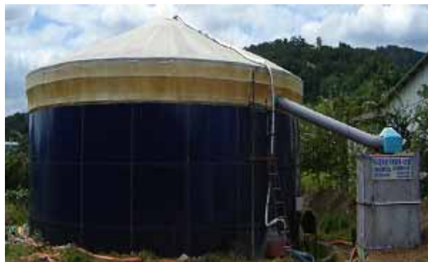
Fig. 11 Offensive odor emitting facility for manure tank
